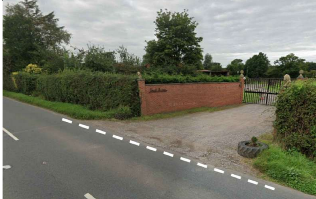
Example of Edge of Carriageway marking across entrance
