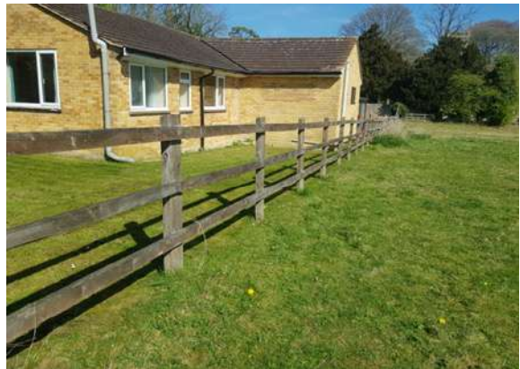
Photo 4: Timber post fencing to western boundary
